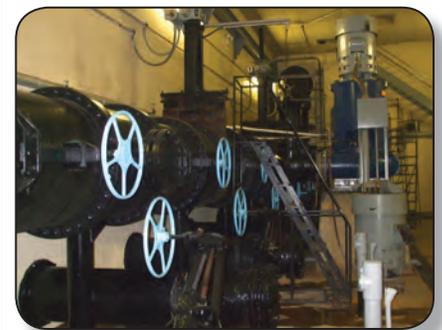
*Fourth level down of the Administration Building where the main interceptor pipe enters the plant (left). Pumps (right) lift the wastewater to the Mixing Well where the treatment process begins.*
