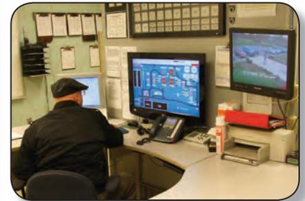
*Control Room in the Administration Building where the processes in the plant are monitored and controlled.*
