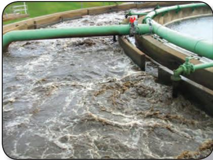
*Primary Clarifier Tank where aeration separates sewage and microbes digest the sludge in the outer ring. Sludge is deposited in the quiescent waters of the center ring.*
