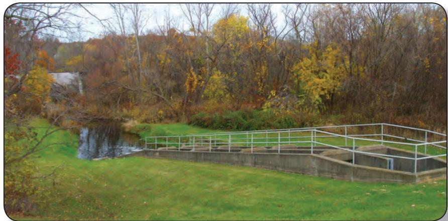
*Outfall structure on French Creek at the end of the treatment process, where up to 5 million gallons of water are discharged to the creek each day.*
