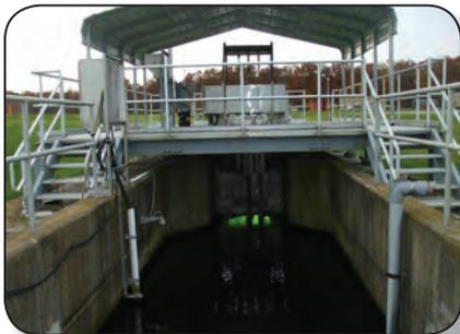
*Automated ultra-violet rays disinfect the processed water as it is discharged from the plant.*
