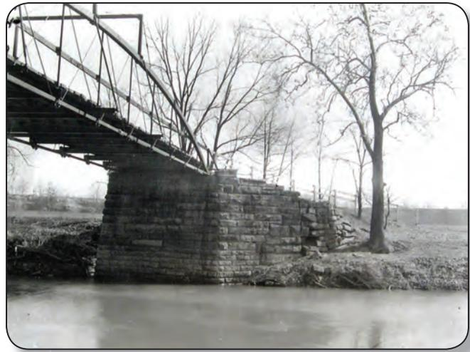
South abutment to Days Dam steel-truss bridge (~1910). The Black River flows under the bridge here, but has since abandoned this meander channel (Black River Historical Society).
