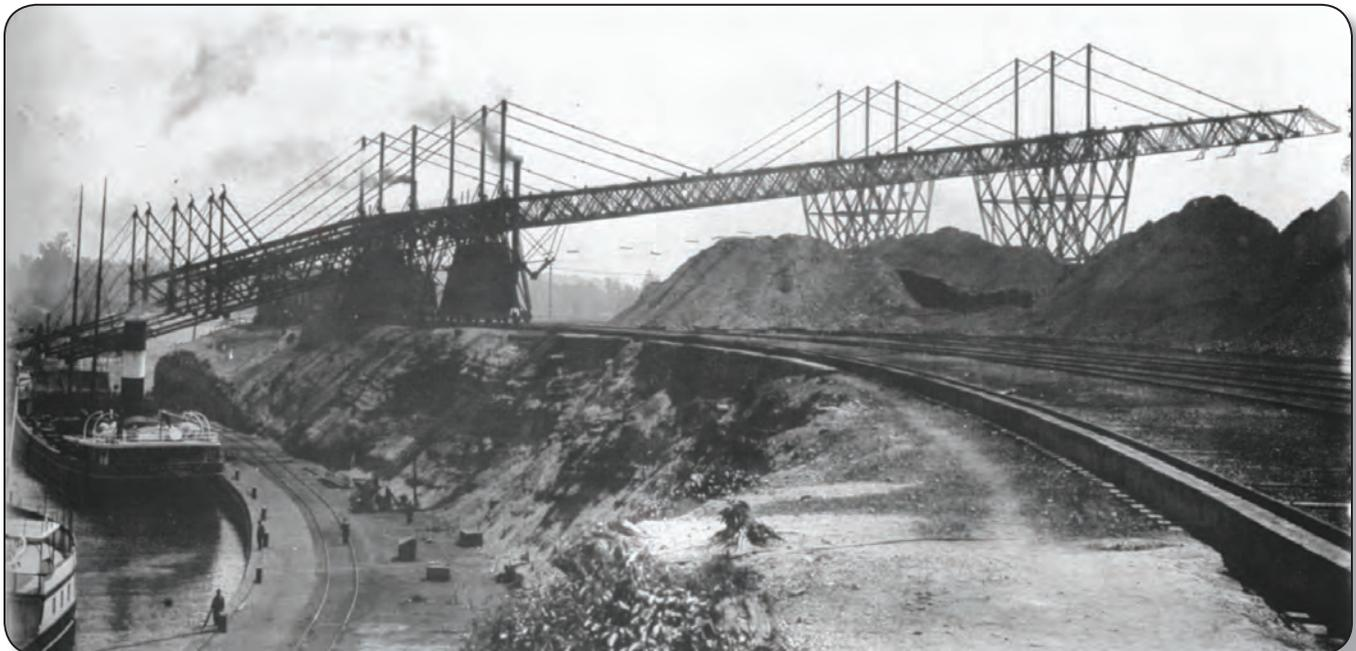
*McMyler hoist ore unloader at the steel mill dock on the Black River (circa 1900).*
