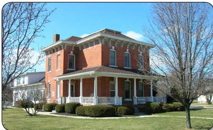
Saint Teresa Parish House
