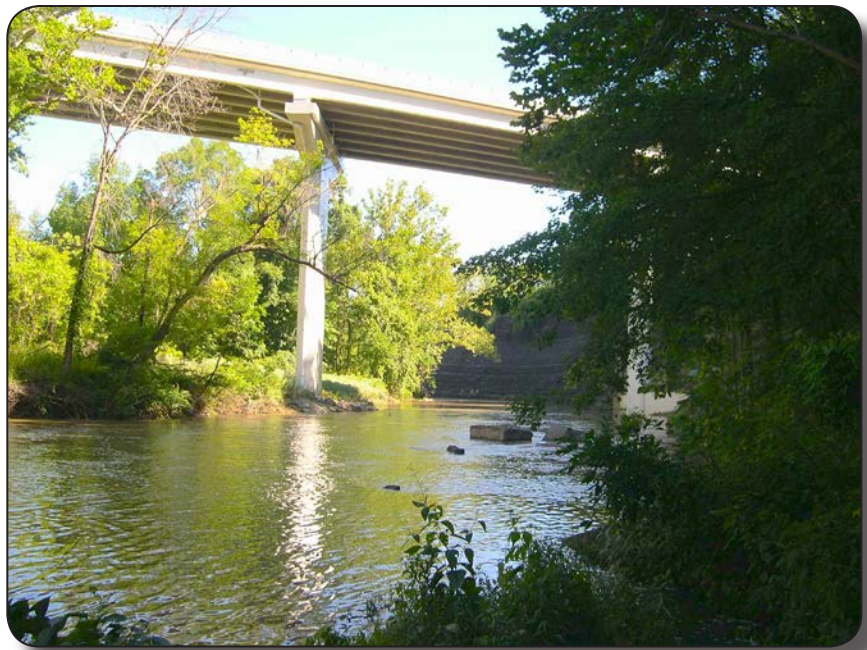
New viaduct bridge, 2003
