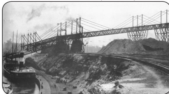
McMyler hoist ore unloader at the steel mill dock on the Black River (circa 1900)
