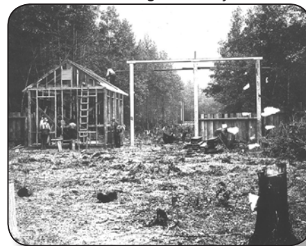
Construction of the steel mill's Pearl Avenue gate in July 1894
