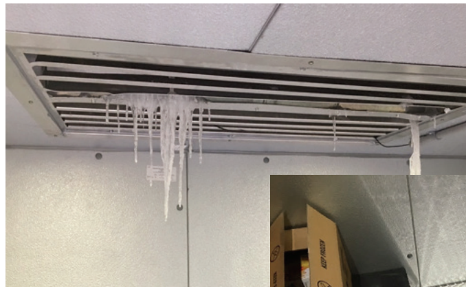
Figure 1 - Ceiling Before with Digital Controller
