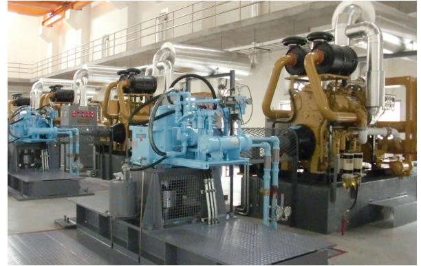
The Logan LC318 Bell-Housing PTO clutches provide on-demand power to the Flender gear boxes that run the pumps
