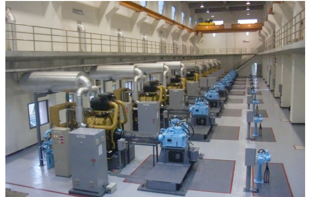
The Jingmei pumping station uses a lineup of CAT engines with Logan Bell-Housing PTO clutches to power their pumps
