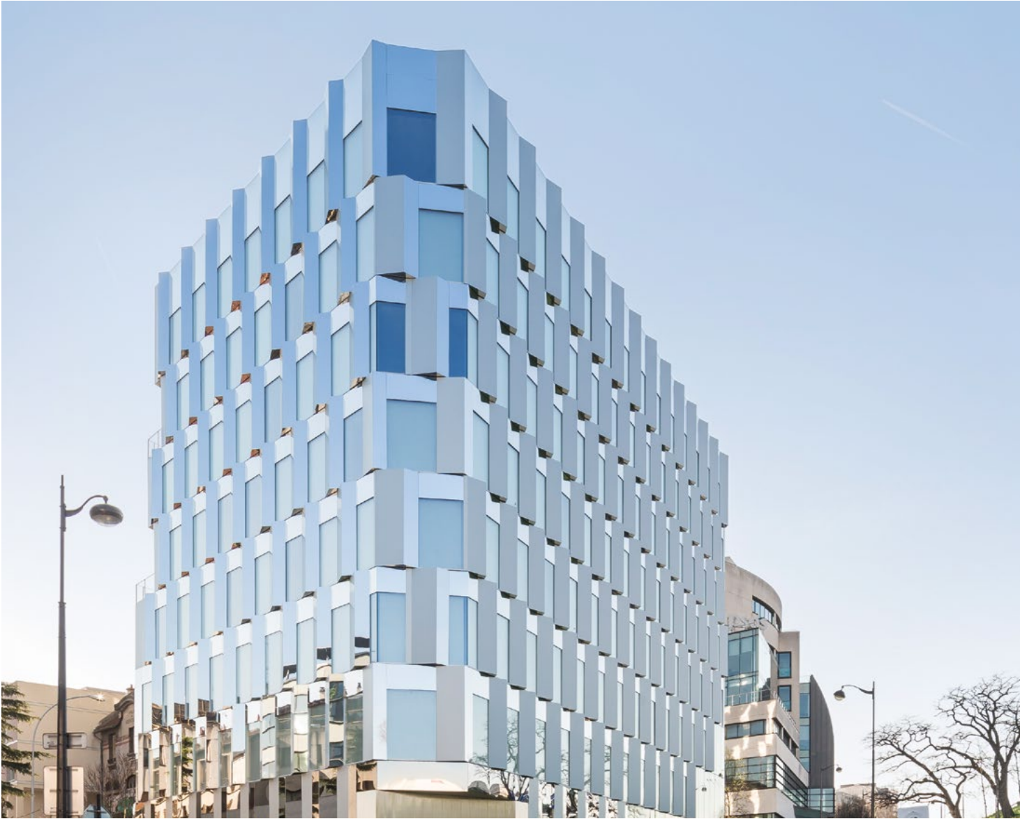
©Sergio Grazia Riverside Gently in France. Facade made of DECO PRIME®4 with FL01
